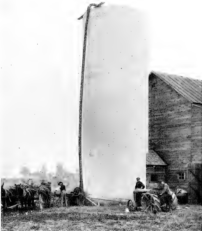
FIG. 250.—Tractor running a silage cutter and blowing the cut corn into a very high concrete silo. (Tennessee Power Farming Review.)
